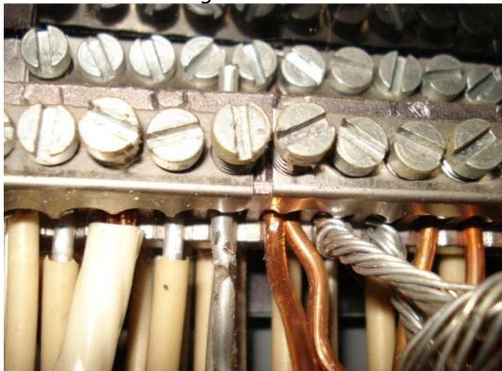
Neglected connections in outlets, switches and light fixtures containing aluminum wiring become increasingly dangerous over time. Poor connections cause wiring to overheat, creating a potential fire hazard. In addition, the presence of single-strand aluminum wiring may void a home's insurance policies. Inspectors may instruct their clients to talk with their insurance agents about whether the presence of aluminum wiring in their home is a problem that requires changes to their policy language.
