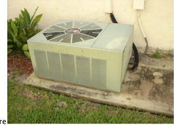
coils of pipe that are surrounded by thousands of thin metal "fins" that allow the coils more surface area to exchange heat. Follow these tips when cleaning the exterior condenser unit and its inner components — after turning off power to the unit!
