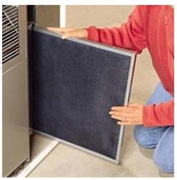
energy costs and reducing energy efficiency. The filter should be replaced monthly during heavy use during the cooling seasons. You may need to change the filter
